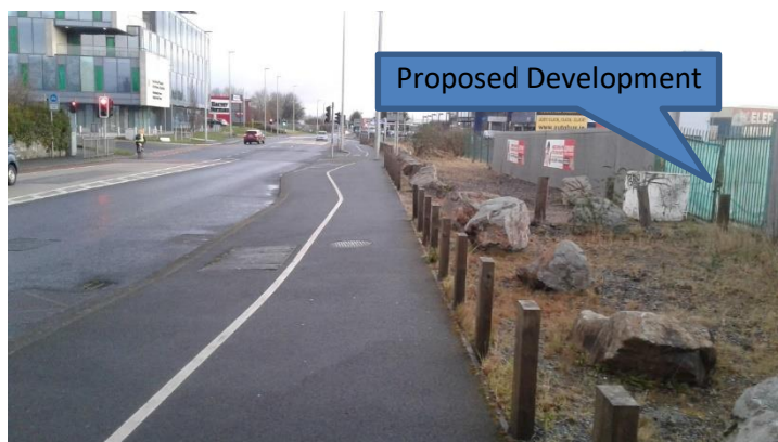
Plate 3.2 – Existing Pedestrian Facilities at Greenhills Road /Airton Road Junction
